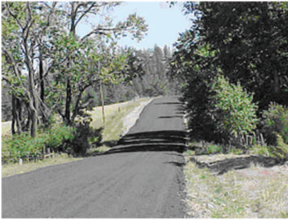
Montana pugmilled and grader placed RAP.
