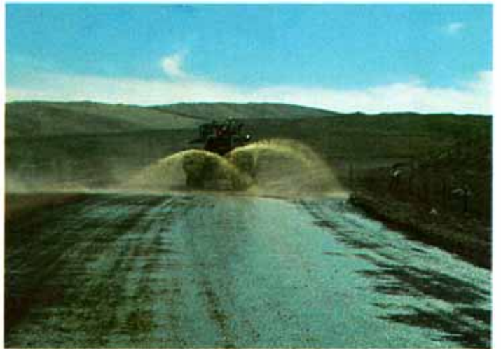
Coherex being sprayed on haul road at Bridger Coal, Wyoming.
